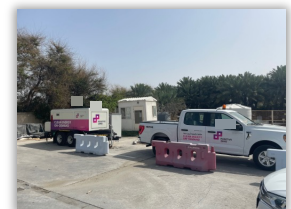
430kWh Battery Container and 250kW Discharging Station
