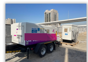
430kWh Battery Container and 250kW Discharging Station
